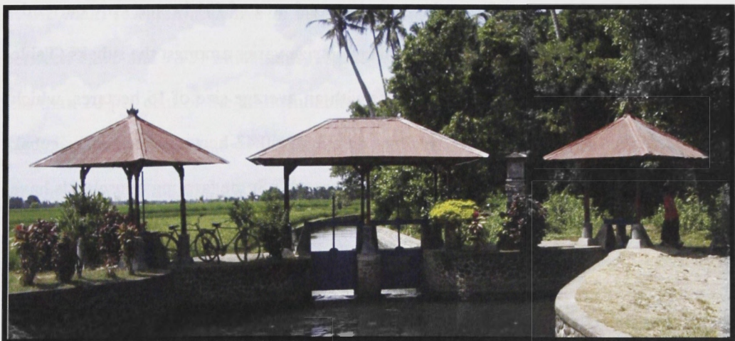
Figure 4.3: Gated diversion weirs: subak Aban (left), subak Dukuh (right)
