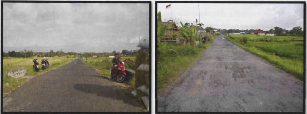
Figure 6.19: Road development on the Anggungan side, 2007 and 2009
